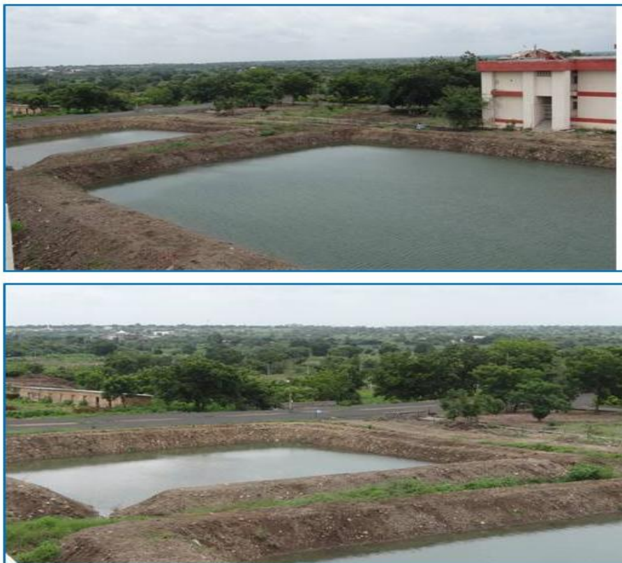
Figure 2 Water tanks at SRTM University Campus
